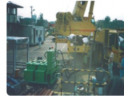
Petrochemical (Ulsan SK Oil Refinery)
