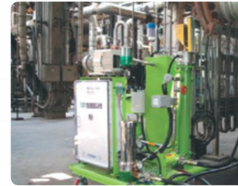
Petrochemical (Ulsan SK Oil Refinery)
